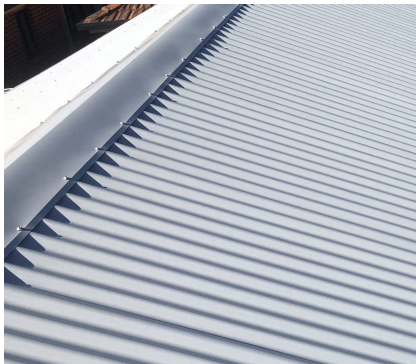
CR Colorbond custom orb roofing Colour: White
